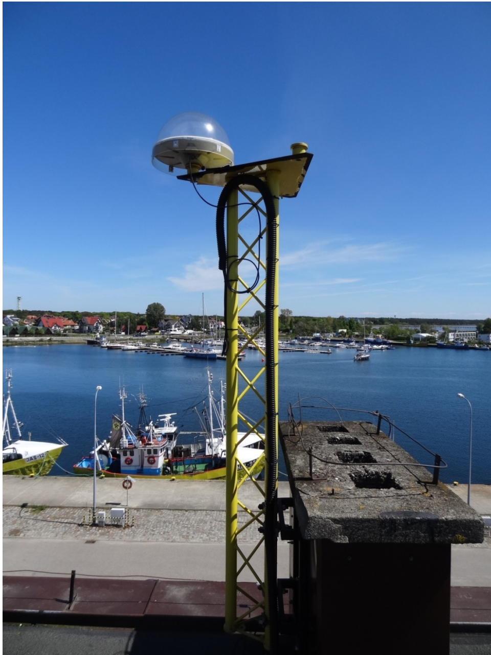
Figure 2-6: View from the roof of the Jastarnia harbor. In the foreground, the RTK station mast, which can be used to mount the rod antenna of the VDES receiver. Two additional RF cables were led to it.
