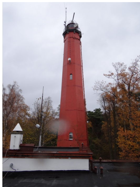
Figure 2-3: The Hel Lighthouse and the roof of the engine room with the antenna of the RTK station.
