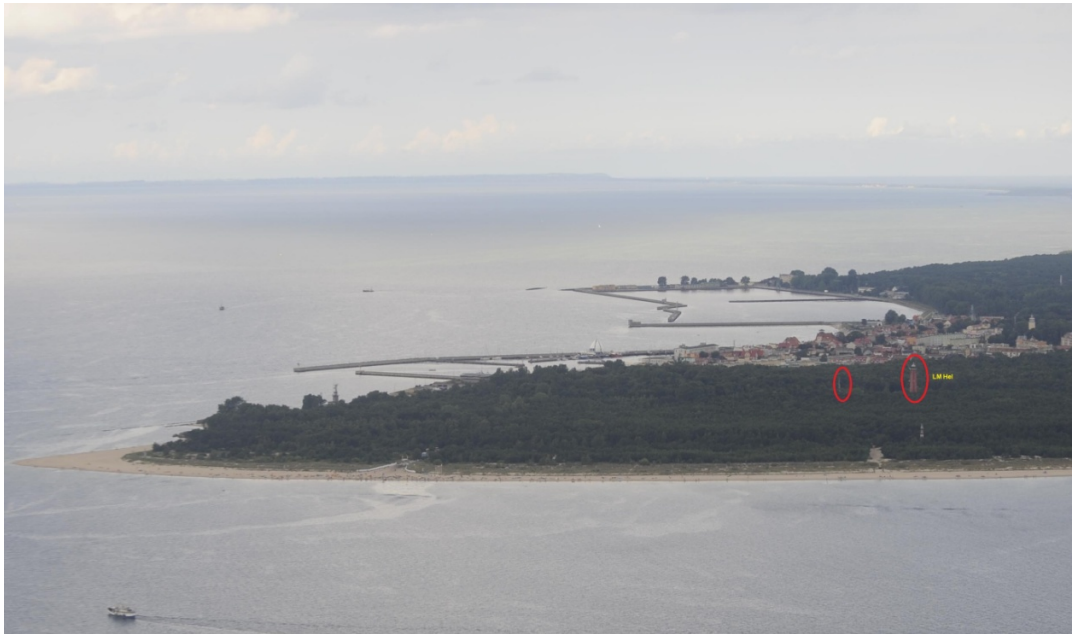
Figure 2-2: Location of the Hel Lighthouse in relation to the Gdańsk Bay water line towards Gdynia.
